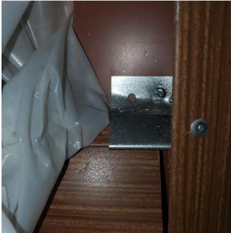
Photo No. 3 Failure Photo #2
