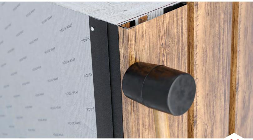
Once the trimmed Random Plank is in place and secured, you can install the Top J Insert. With a mallet or non-marring object gently tap into place, ensuring not to scratch or damage the J.
