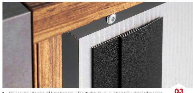
• This image shows the measured & cut Starter Strip sliding into place. Ensure your Starter Strip is aligned tightly against the material your Random Plank is starting next to (for this install, we're starting next to a stucco wall), or against the wall where the Random Plank will be installed.
