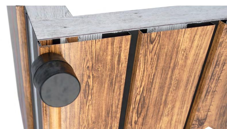
Once the trimmed Random Plank is in place and secured, you can install the Top J Insert. With a mallet or nonmarring object gently tap into place, ensuring not to scratch or damage the J.
