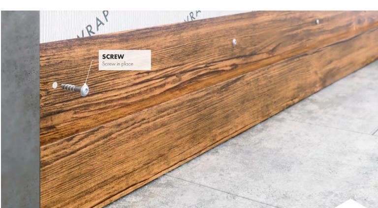
Fasten the Box Base over the U-Support using the appropriate fasteners for wood or steel. Fasten the Box Base to the substrate studs.
