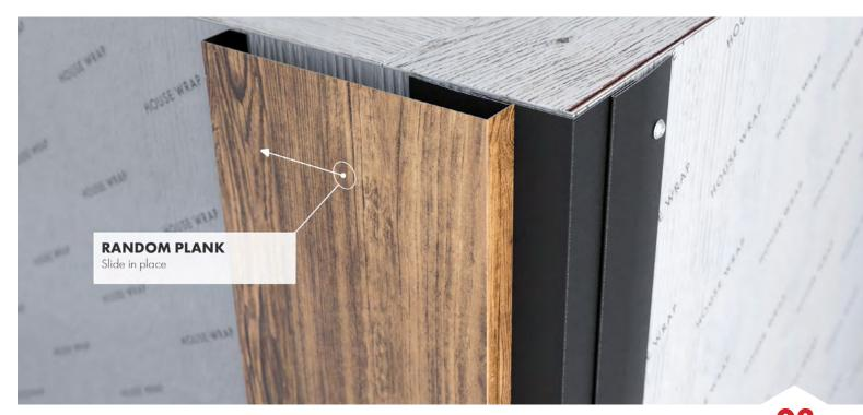
• After your OS Starter Strips are installed, slide your first Random Plank into place. In this case, you will pull or push the Random Plank snug against the inside of your Starter Strips.
