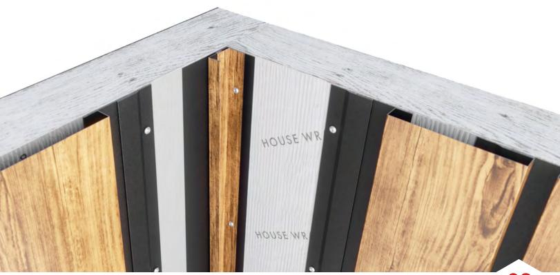
• Next, measure & cut your Two-Piece J-Channel to the same height as the L-Trim in the previous step. You can cut the J using one of the methods in the cut guide shown at the beginning of this guide. Once the Two-Piece J is cut, place over the Inside L-Trim, and slide the J insert out of the bottom J receiver.
