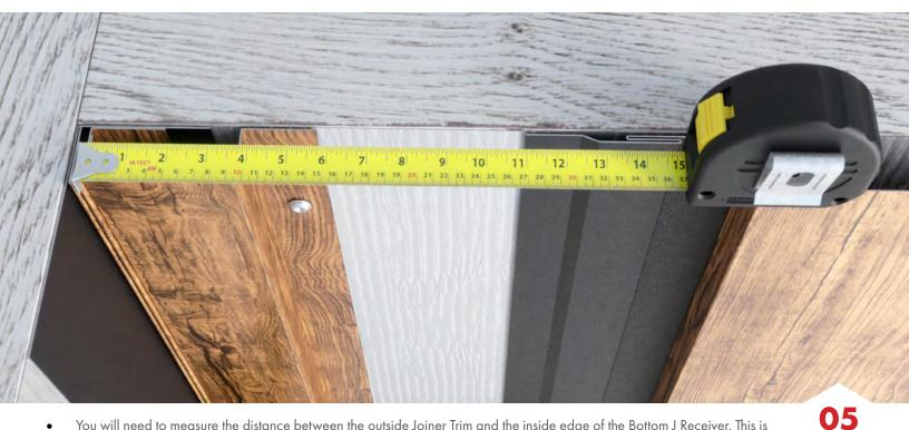
You will need to measure the distance between the outside Joiner Trim and the inside edge of the Bottom J Receiver. This is the distance your trimmed Random Plank will need to cover.
