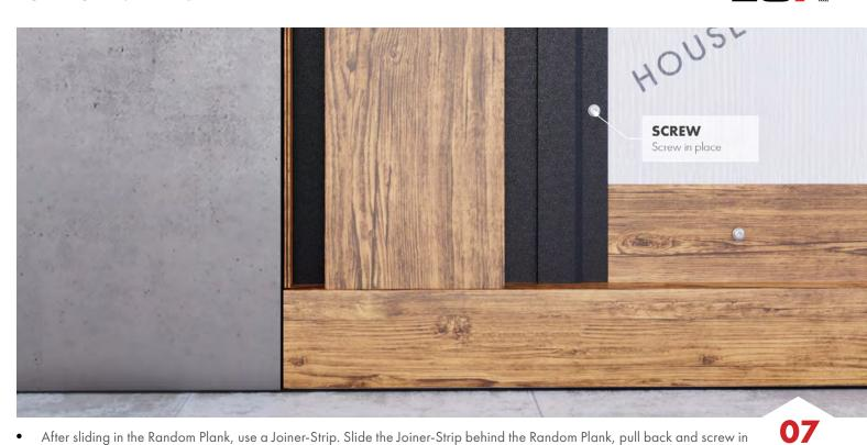
• After sliding in the Random Plank, use a Joiner-Strip. Slide the Joiner-Strip behind the Random Plank, pull back and screw in place. Never pull back too tightly; panels need to be able to expand and contract.
