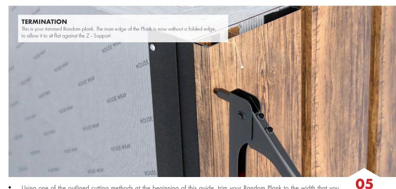
• Using one of the outlined cutting methods at the beginning of this guide, trim your Random Plank to the width that you measured in the previous step. The trimmed Random Plank then slides into the hem on the end of the last Joiner Trim and sits flat against the Z-Support. The Random Plank is then fastened using stainless steel rivets.
