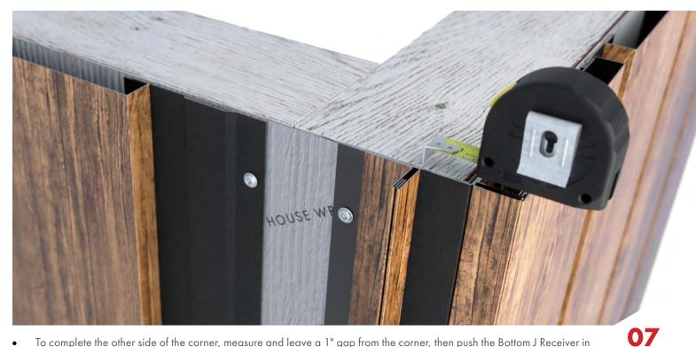
• To complete the other side of the corner, measure and leave a 1" gap from the corner, then push the Bottom J Receiver in firmly and fasten to the substrate with the appropriate wood or metal screws. Ensure you screw through both layers of the Bottom J Receiver and the L-Trim.
