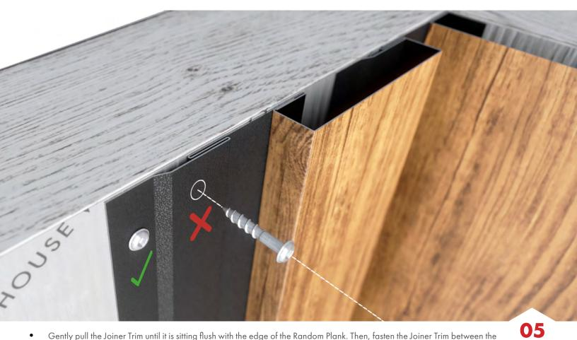
Gently pull the Joiner Trim until it is sitting flush with the edge of the Random Plank. Then, fasten the Joiner Trim between the hems with the appropriate screws. Be cautious not to screw through the hem that the next Random Plank needs to slide into.
