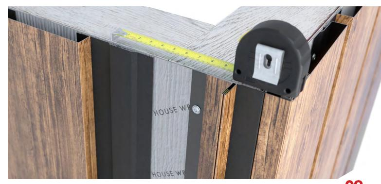
• Next, measure the distance between the exposed Joiner Trim and the inside edge of the Bottom J Receiver. This is the distance your trimmed Random Plank will cover. Using any one of the outlined methods in the cutting guide at the beginning of this guide, trim your Random Plank to the correct width.
