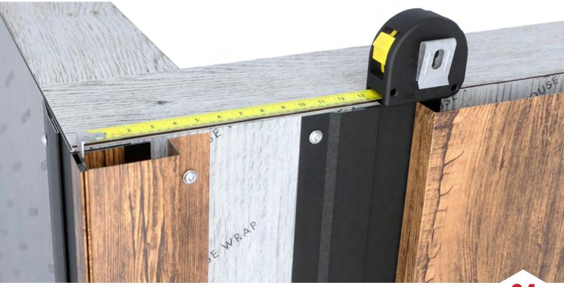
Measure the distance between the exposed Joiner Trim hem and the inside edge of the Bottom J Receiver. This is the distance
