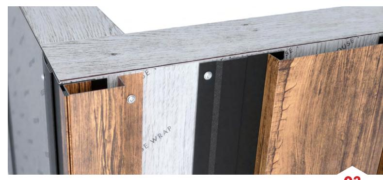
• The next step is to measure, cut, and attach the Z-Support. This trim is used as a supplementary support for the Random Plank as you will need to trim the Random Plank edge to ensure it cleanly ends in the corner. Push the Z-Support firmly against the Bottom J Receiver and fasten to the substrate with the appropriate wood or metal screws.
