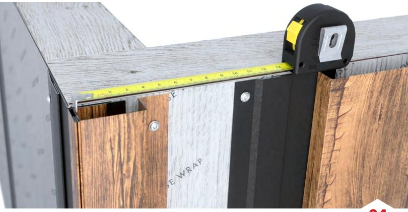
Next, measure the distance between the exposed Joiner Trim and the inside edge of the Bottom J Receiver. This is the distance
